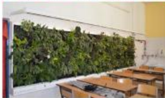
Fig. 3. Living wall system in the greened classroom.
